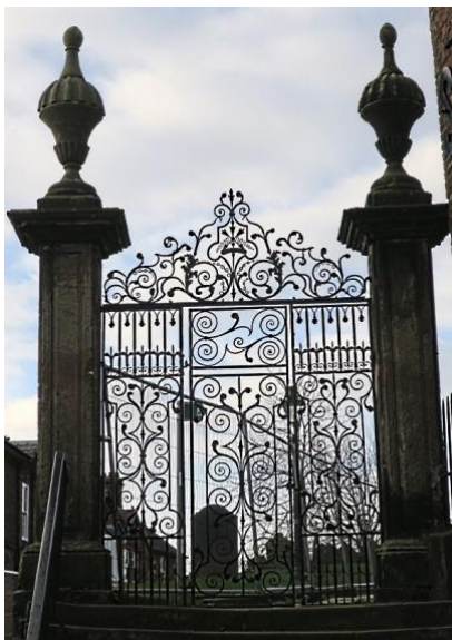
Gate and piers in the SE corner of the churchyard
